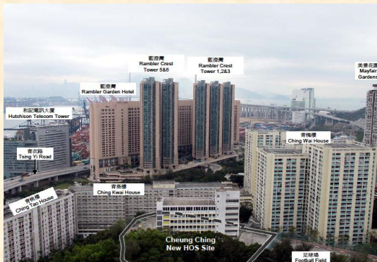
Ching Hong Road, Tsing Yi 青衣青康路
