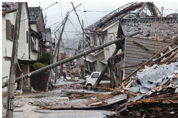
Houses destroyed by the earthquake in Kawai-machi, Wajima, Ishikawa Prefecture
